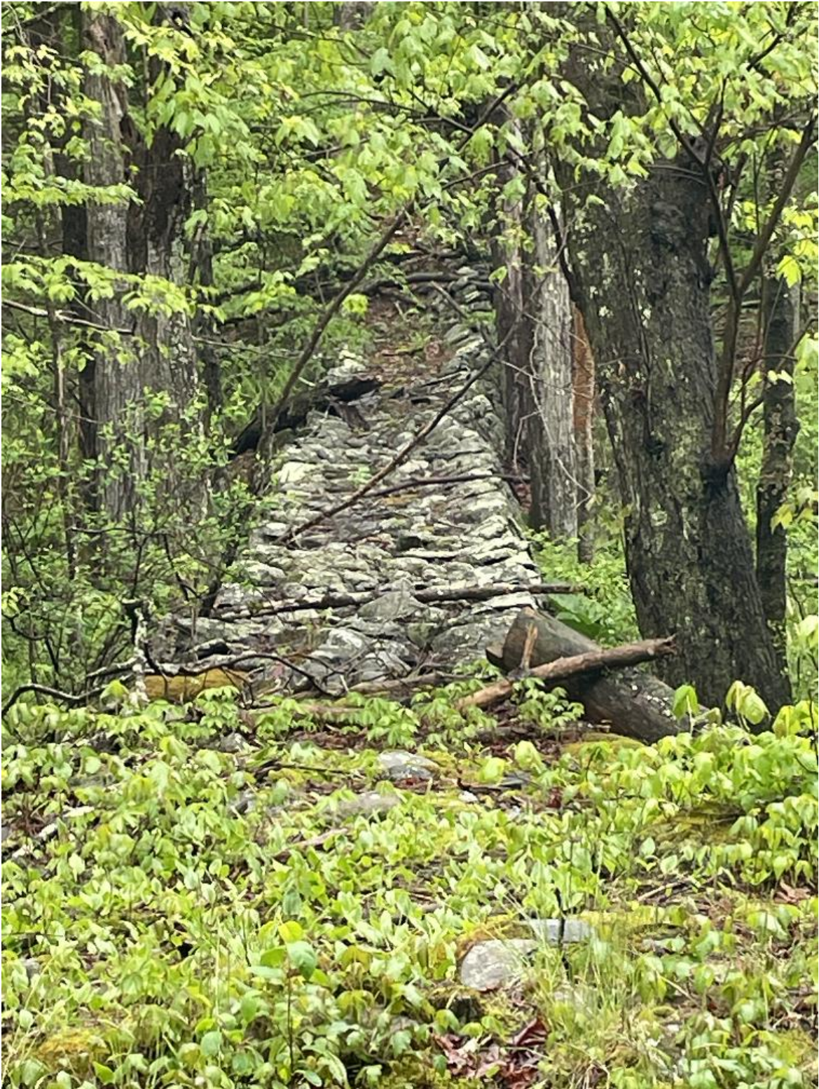
A view of one of the Stone walls as seen from Pasay road on the north side of the house foundation:
